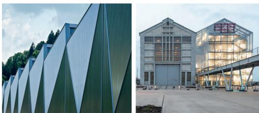
Cladding might be arranged in an angular format to create texture and interest. North facing rooflights allow natural light to penetrate the plant and limit the requirement for artificial lighting.
