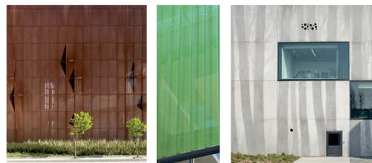
Mesh cladding would allow views through to the plant inside, using Cor-Ten steel would reflect the previous steelworks on the site. Hues of green mesh or cladding could be added, influenced by the surrounding landscape and would provide contrast with the rusty rich brown of the Cor-Ten.
